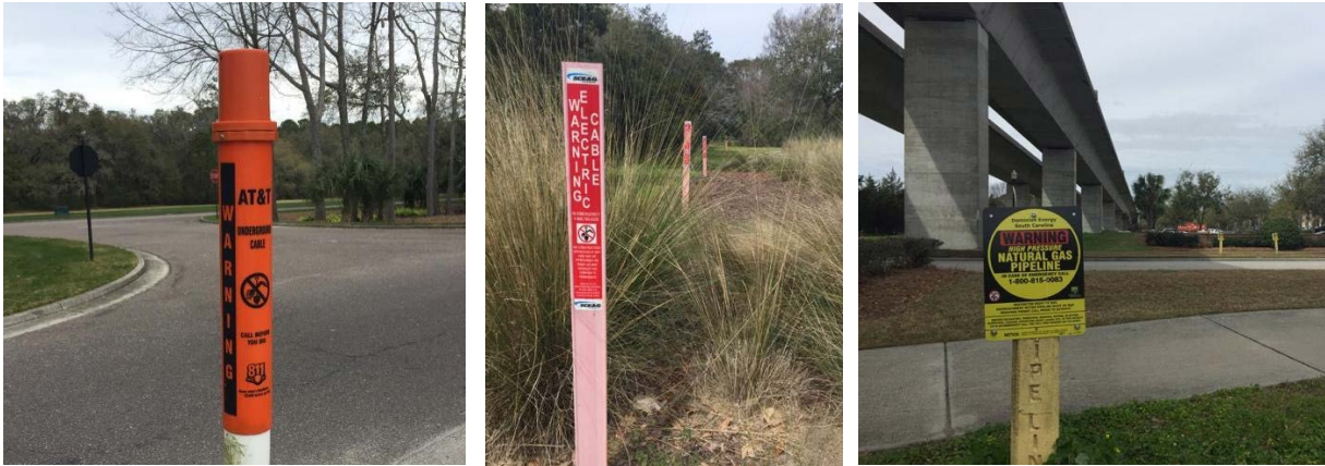
Examples of permanent warning signs for awareness and protection of underground facilities.
